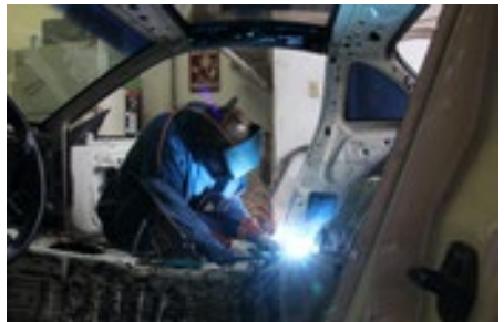
Car production and repair shops
